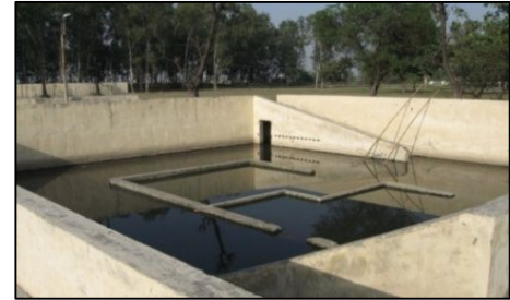
Fig no.89: Disposal Work, Fatehpur
