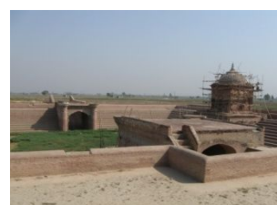
Fig no.50: Pul Kanjri under renovation
