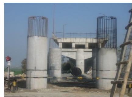
Fig no.81: ROB under construction
