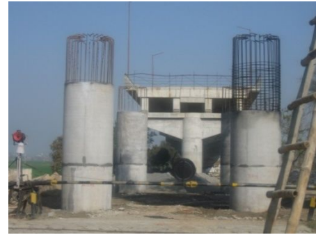
Fig no.84: ROB at Aproach road to Baba Bakala Under progress
