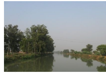
Fig no.110 UBDC (1) near Mehta road
