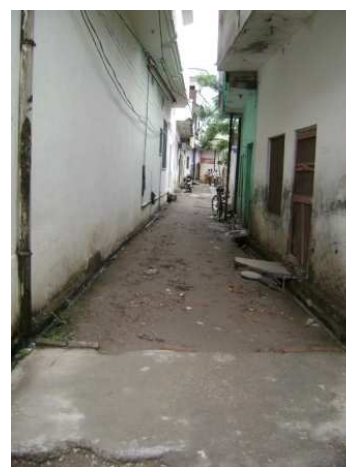
Fig no.24: Open Drains within slum colonies
