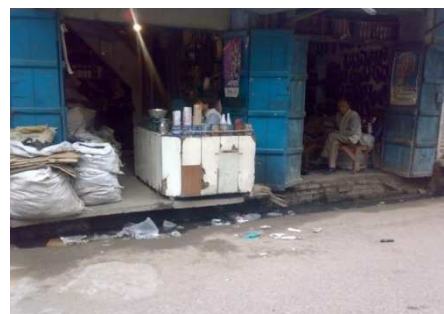
Fig no. 38: Open Drain in Town
