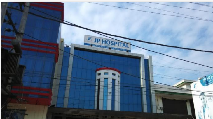
Figure 9 Multispecialty JP Hospital in Zirakpur
