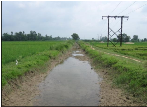
Fig. 49: Back Water in Batala Distributary
