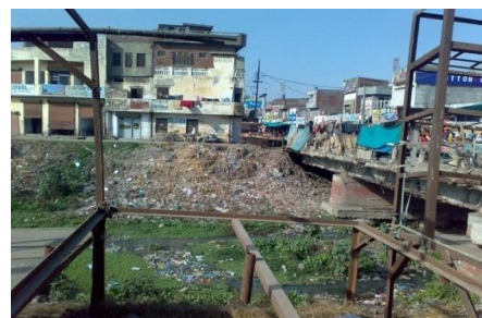
Fig. 35: Open Dumping of Garbage at Hathi Gate
